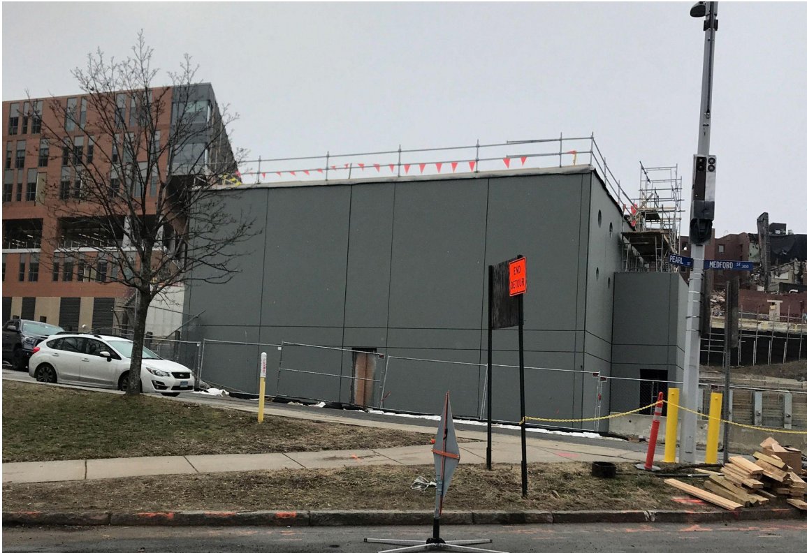
TPSS BUILDING, NORTHEAST FACE, MEDFORD STREET (AND PEARL STREET)
