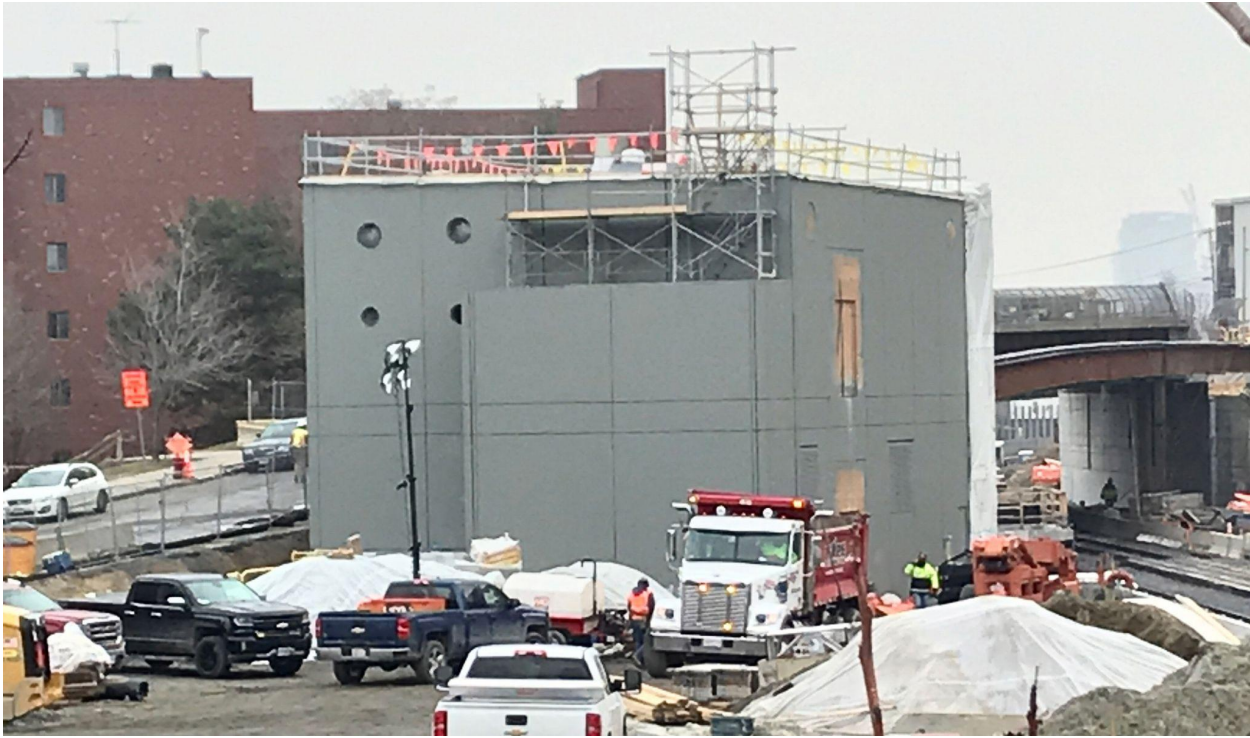
TPSS BUILDING, SOUTHWEST FACE (WITH MEDFORD STREET BRIDGE IN BACKGROUND)
